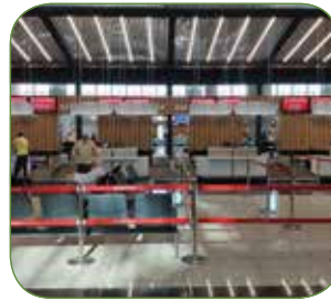
Figure 3. FFU placed over the airport check-in counters
